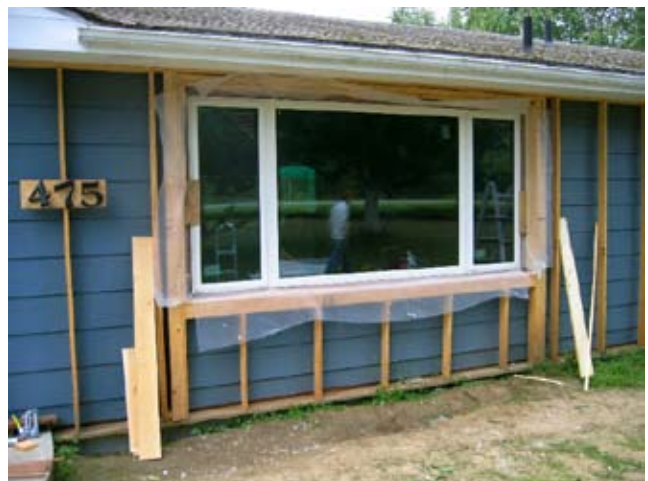
Figure 2. A photo by the author of his own house retrofit showing both the exterior wall being framed in and a new superinsulated window being installed in the rough opening of the old wall. Both of these are examples of how to retrofit both windows and walls with more insulation and a better performance window. The superwindow is described in the Fall 2005 issue of the Alaska Building Science News . It is a fiberglass framed quad-pane, krypton-fill window, 10 feet wide and 5 feet high with a measured R-value at approximately -20°F of 13.25 over a 36-hour period.
